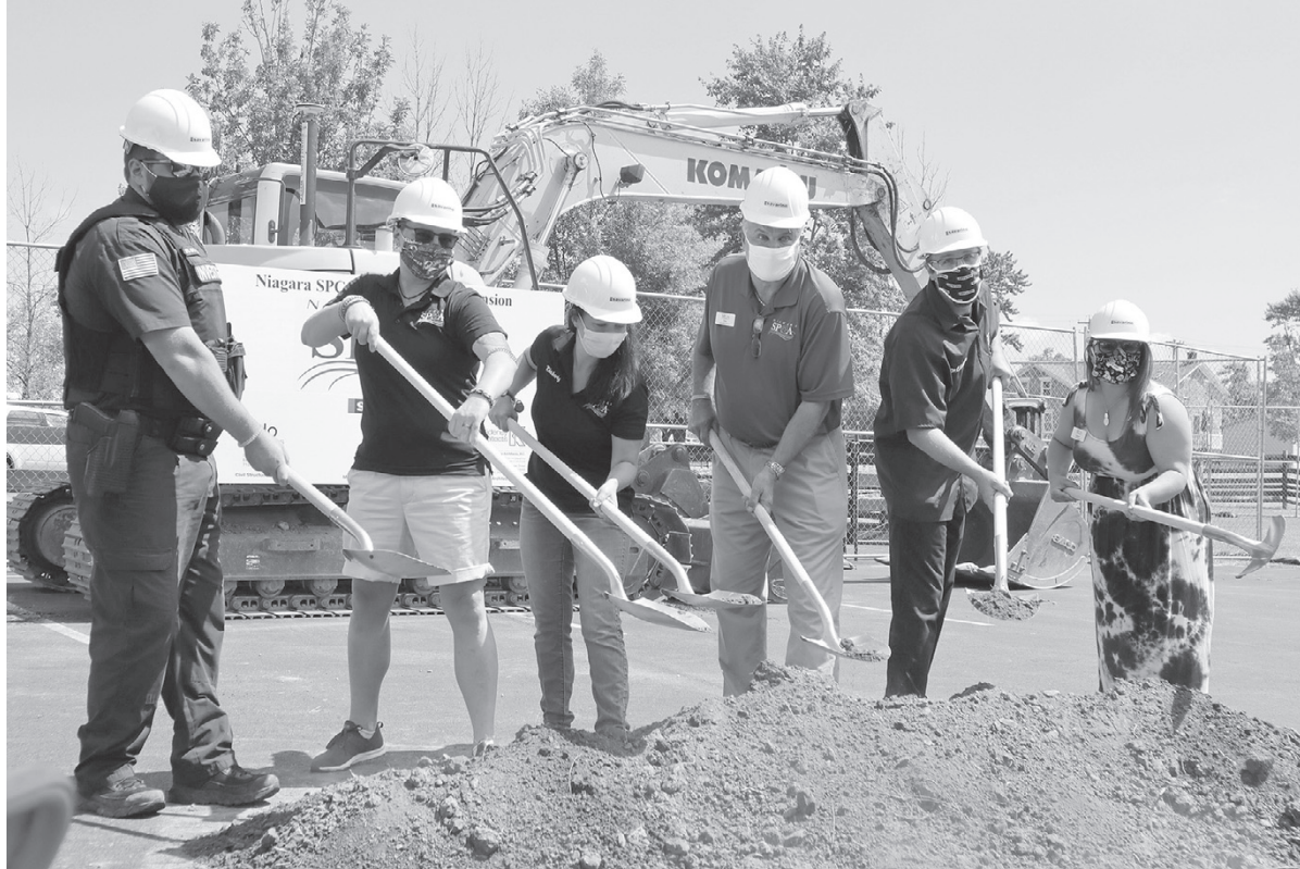
Officials broke ground late last week on a new addition to the Niagara SPCA. (Photo by Michael DePietro)
